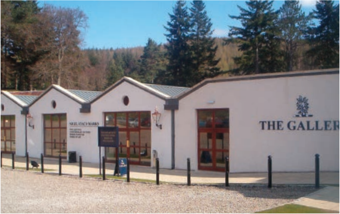
UVF films installed at House of Bruar
