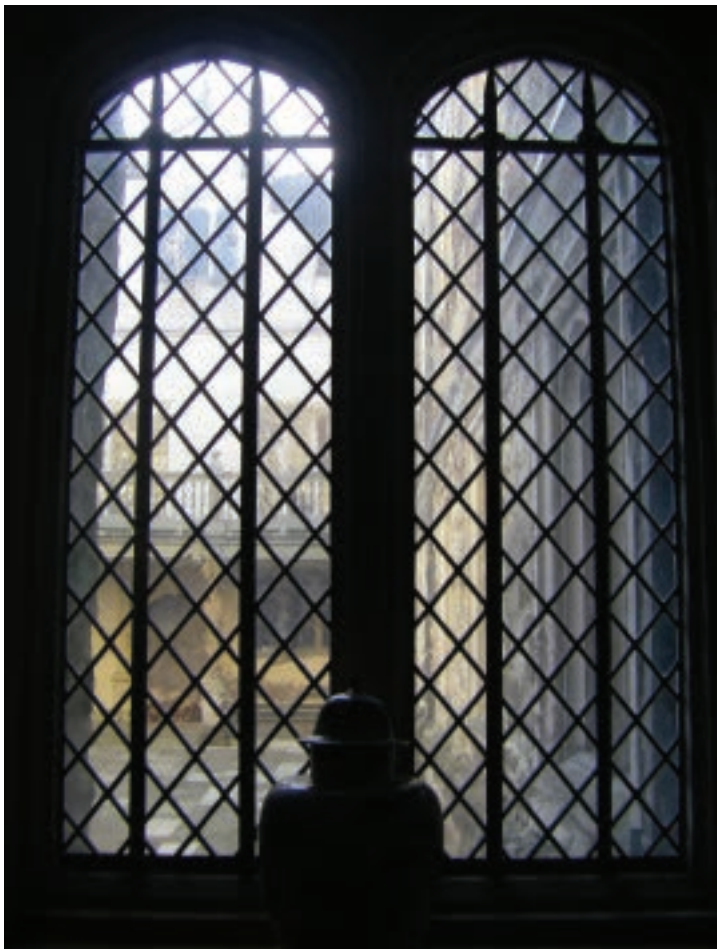
Uvista panels installed at Knole
