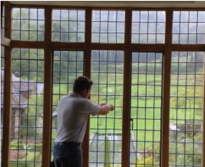
UVX films installed on Leaded Bay (private client)
