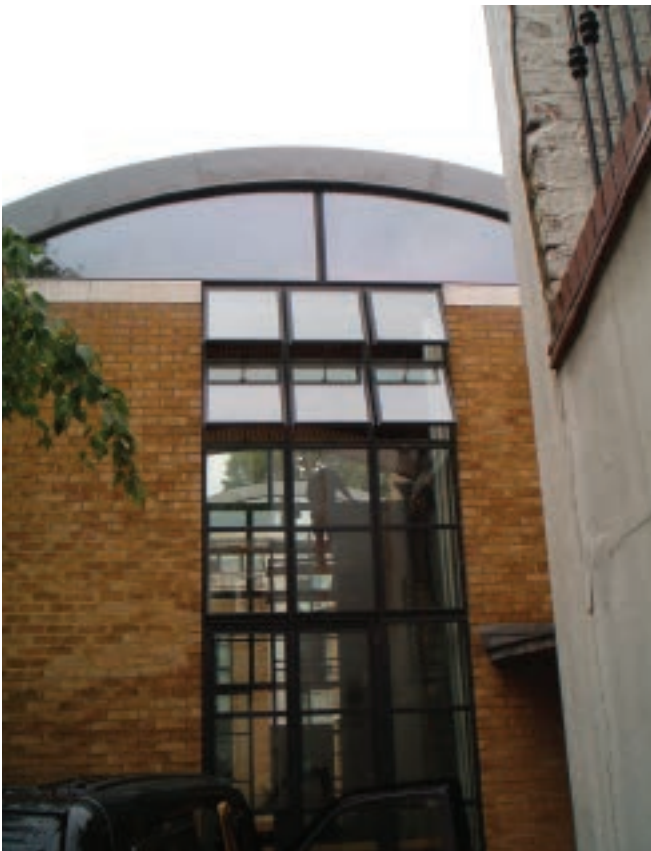
UVX films installation London (private client)
